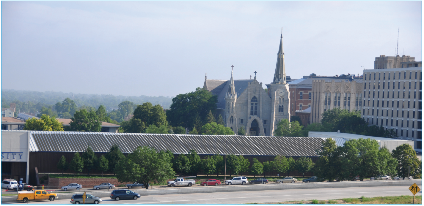
Above: The Kiewit Fitness Center solar roof will provide 20,500 watts of power.
