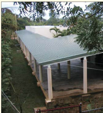
A view from the back of the newly constructed ILAC Health Center.
