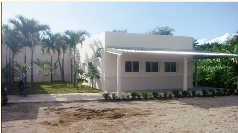
The ILAC Health Center will serve as a modern facility where rural Dominicans can receive medical care.
